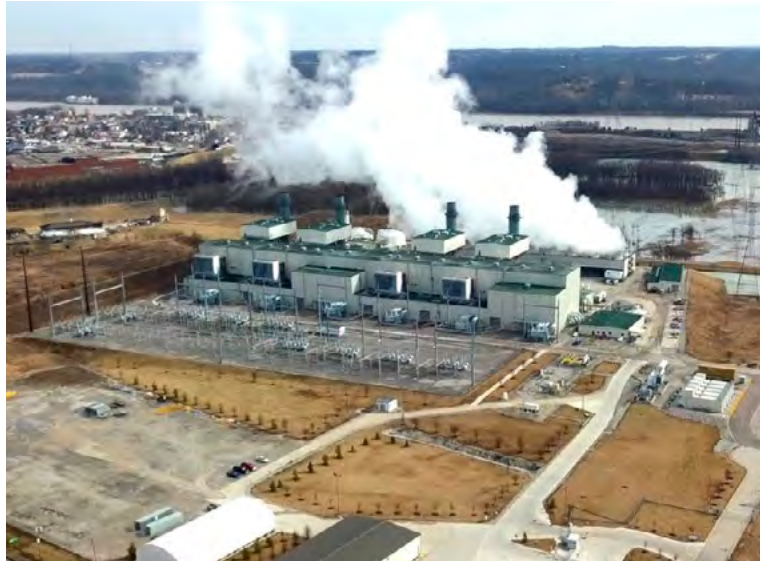
▲ The Lawrenceburg facility is a 1,186MW gas-fired power plant located in Lawrenceburg, Indiana.
