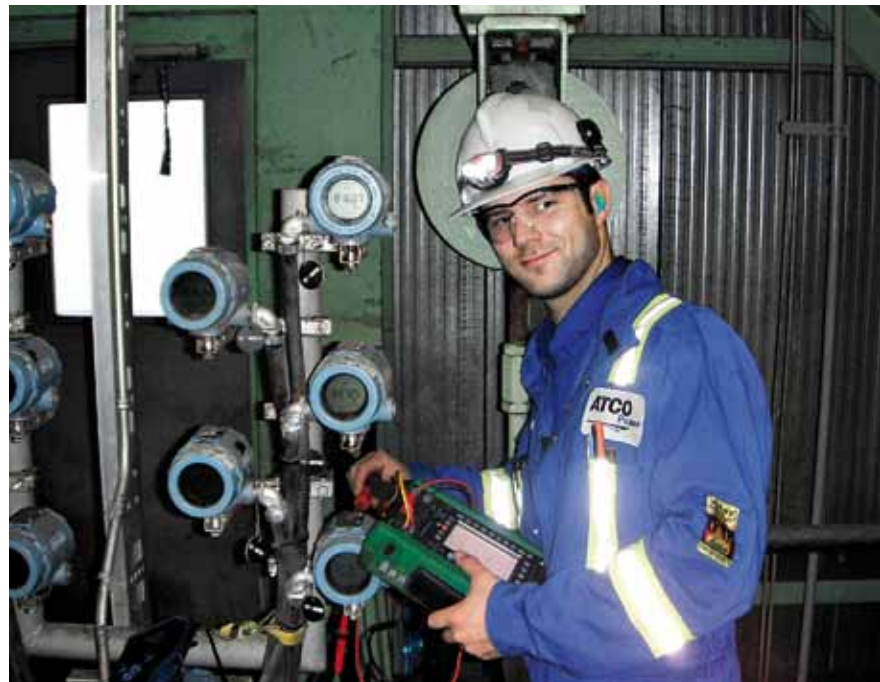
Shane Haugen calibrating a transmitter with MC5.
